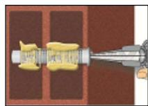
6. Starting from the bottom or back fill the sleeve with adhesive. For quantity of mortar attend cartridges label or installation instructions.
